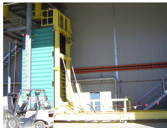
Container loading facility
