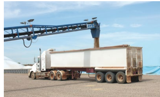
Outloading into truck
