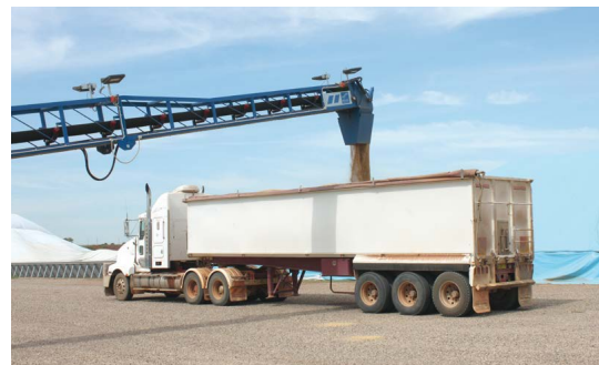
Outloading into truck
