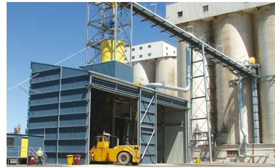
Design and Construct – Container loading facility
