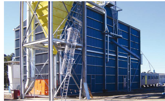
Design and Construct – Container building, structures and complete dust collection system
